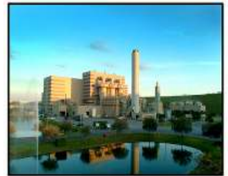
Waste to Energy Resource Recovery Facility
