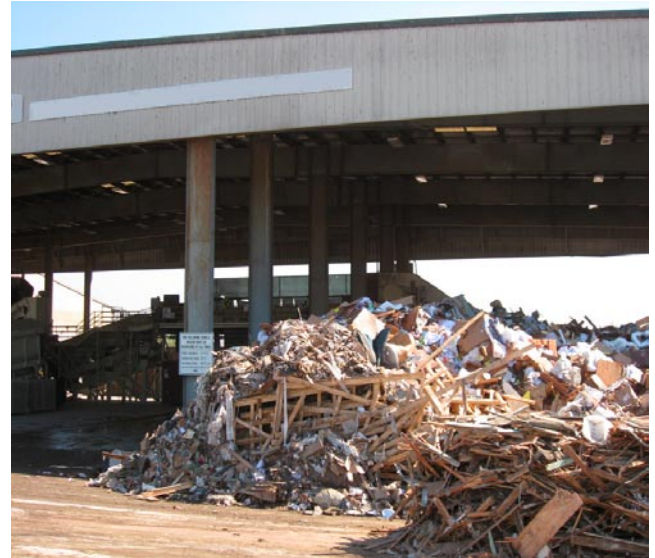
Materials Recovery Facility
