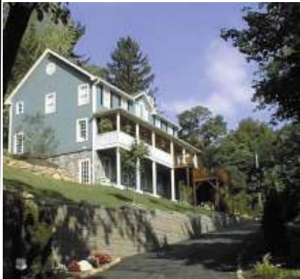
Residential Retaining Wall
