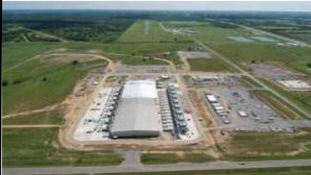
Data Server Facility
